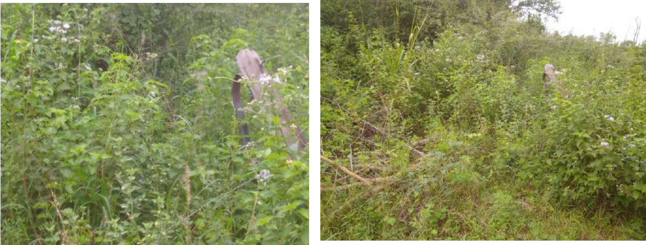
Electric fence broken due to not maintaining properly in Kiul Ara
